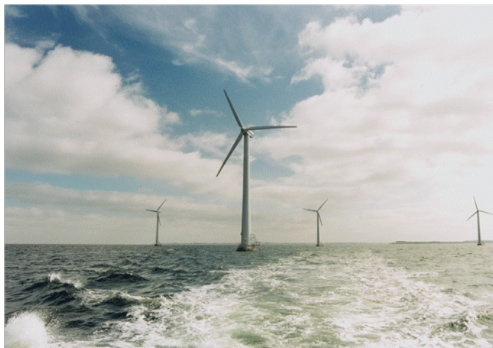
Figure 4.7 Offshore wind farm
