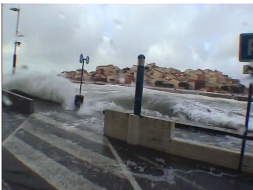
Figure 4.21 Wave overtopping in Capbreton harbour. Upper panel shows a 3D picture of the simulated instantaneous surface elevation in Capbreton entrance channel. Lower panel shows a screenshot of a video taken during the storm on the southern quay of the entrance channel (Source: YouTube, Mars 2014, retrieved from http://www.youtube.com/watch?v=6YuNtXfUHMM )
