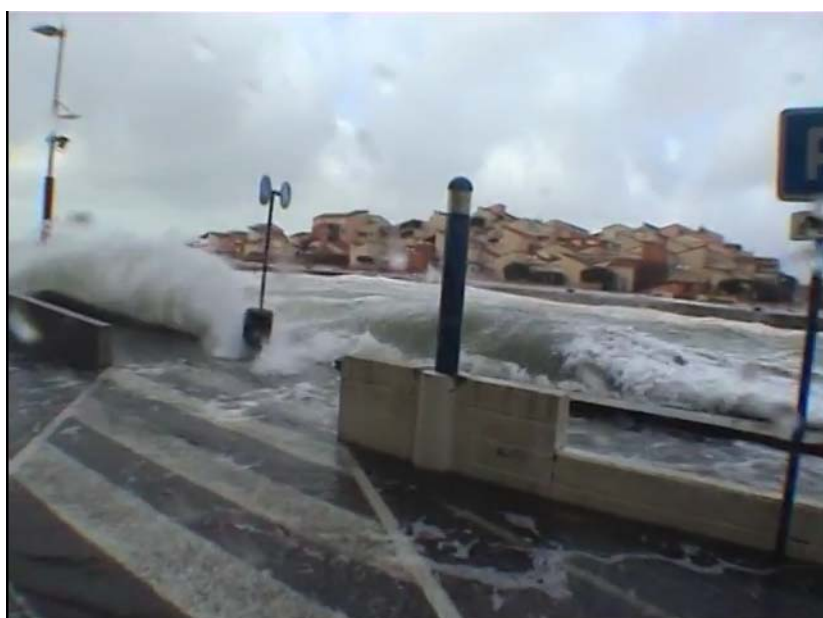
Figure 4.21 Wave overtopping in Capbreton harbour. Upper panel shows a 3D picture of the simulated instantaneous surface elevation in Capbreton entrance channel. Lower panel shows a screenshot of a video taken during the storm on the southern quay of the entrance channel (Source: YouTube, Mars 2014, retrieved from http://www.youtube.com/watch?v=6YuNtXfUHMM )
