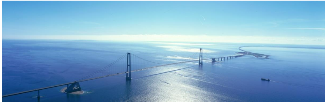
Figure 1.2 The suspension bridge, known as the Eastern Bridge, is a part of the Great Belt Link connection and located between Zealand and Sprogø
