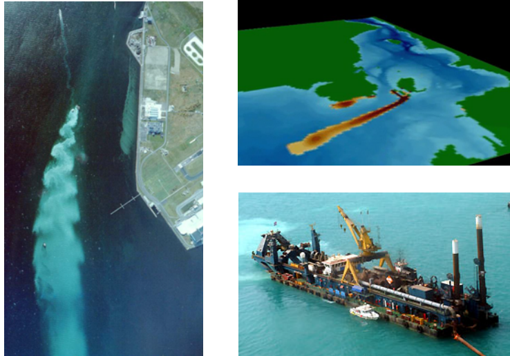
Figure 3.18 Dredging operation in the Sound between Denmark and Sweden. The lower right image shows a photo of Cutter suction dredger Castor
