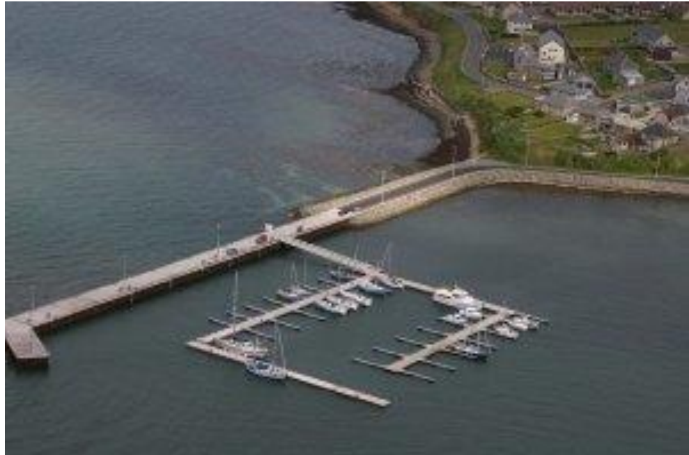
Figure 1.4 Arrangement of pontoons in the Kirkwall Marina, May 2005. Image from http://www.orkneyharbours.com
