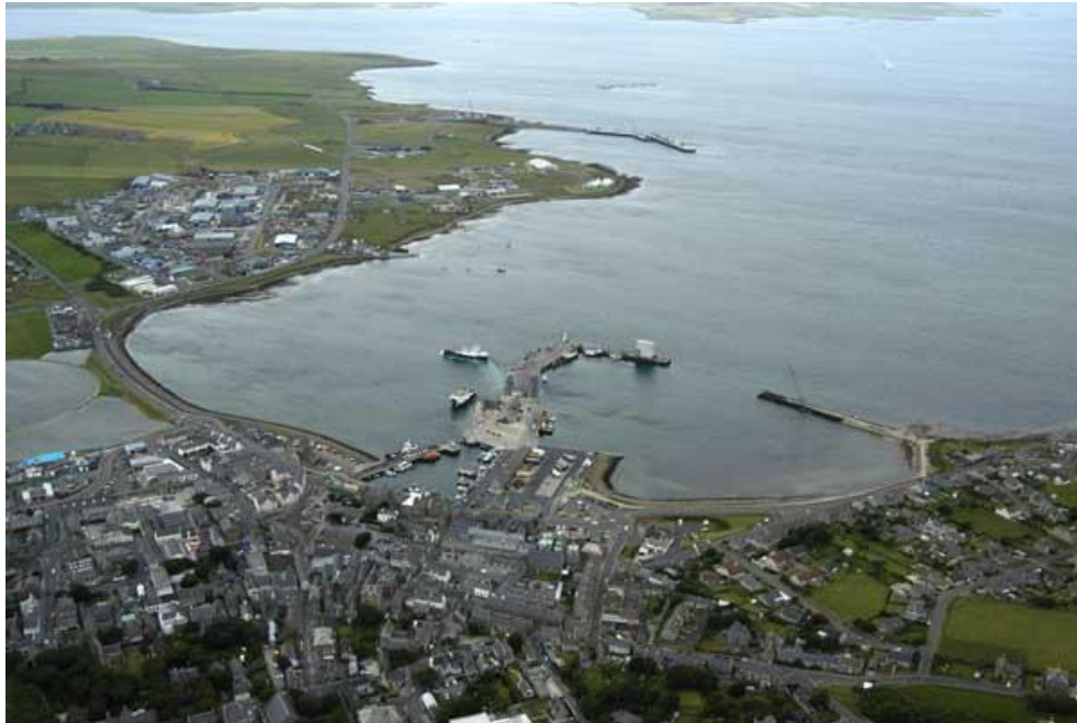
Figure 1.2 Aerial image of the Kirkwall Marina during the construction of the breakwater extension. Image provided by Orkney Islands Council
