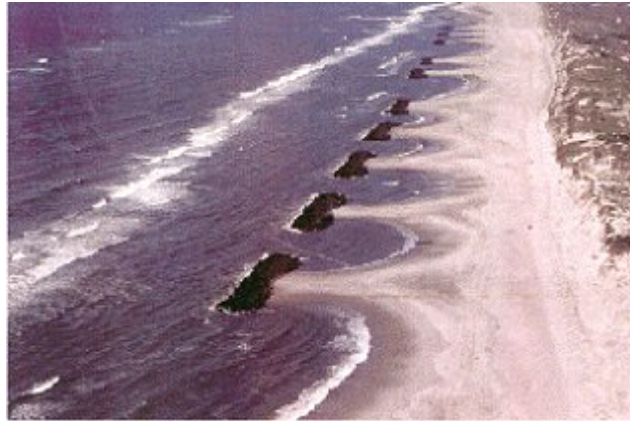
Figure 4.4 Example of detached breakwaters in the coastal zone
