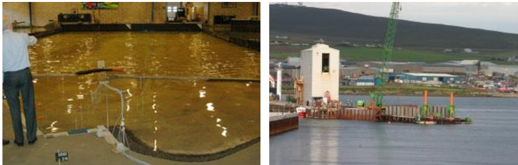
Figure 1.3 Photo of the 3D breakwater model testing at DHI (left panel) and construction of the new breakwater extension (right panel), August 2005. Images from http://www.orkneyharbours.com
